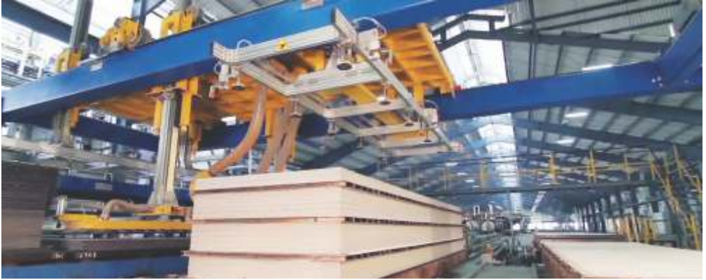
RIL, Keshwana Plant, Kotputli
